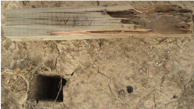
Fig 16- Treated with Celcure samples of E. viminalis , the attack by termites started after 24 month, then the grade No. Reached to 4.6 after 48 month installation in Albaji
