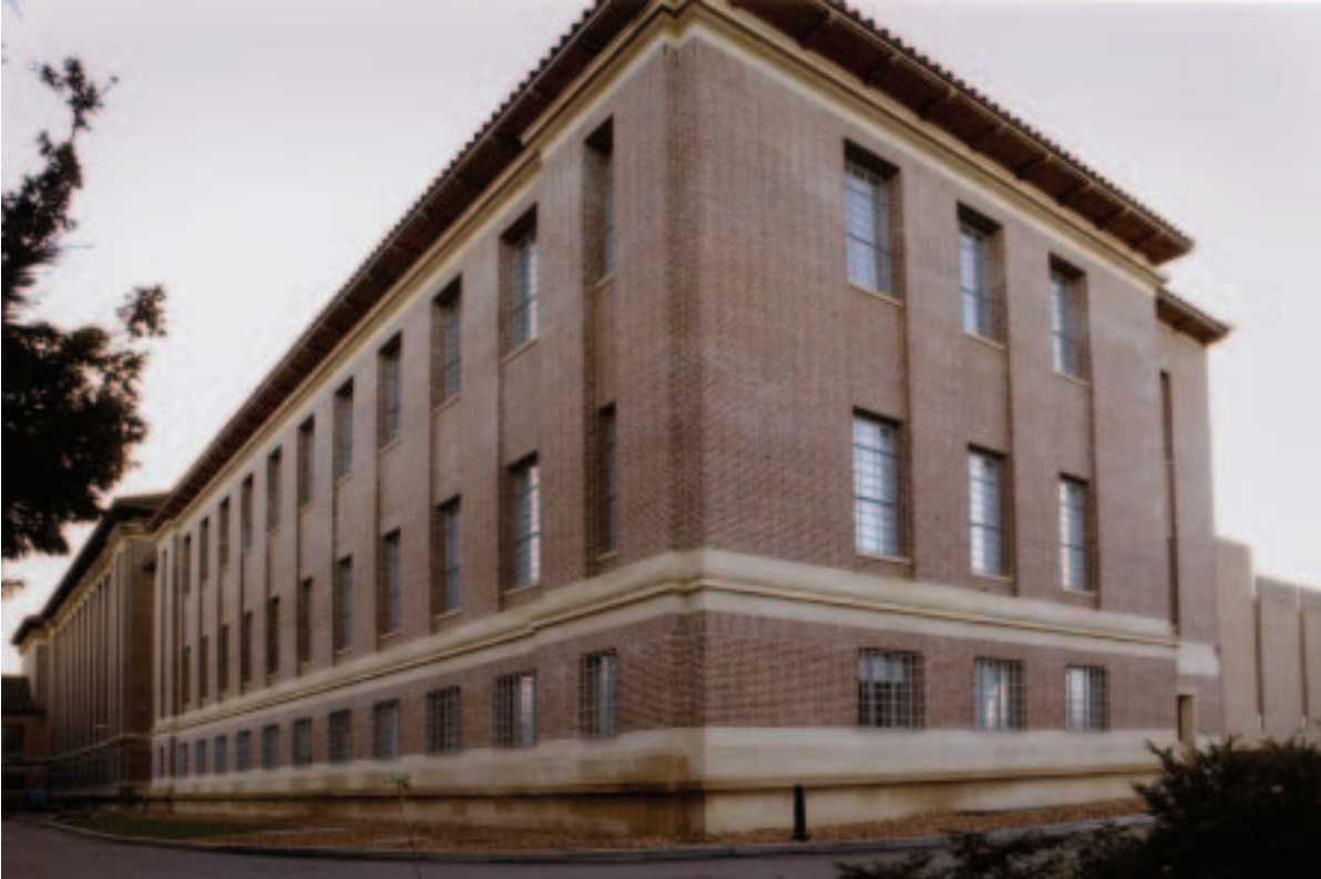
Cambridge University Library, Stage III Extension - Phase 4, North-West Extension , NW Corner, Exterior
