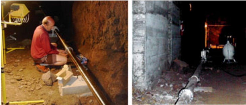
Figure 4. Illustration of the heterogeneously constructed UG2 gyroscope. Many small concrete foundations on the floor of the Cashmere cave support the ring laser structure.
